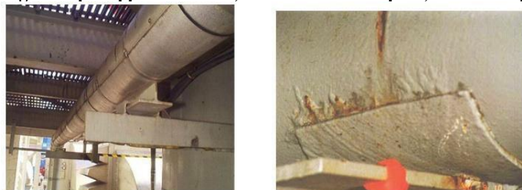
Fig 1.2 Welded supports in pipe
