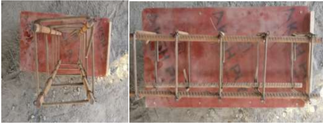
Fig.2 Binding of Reinforcement for square column
