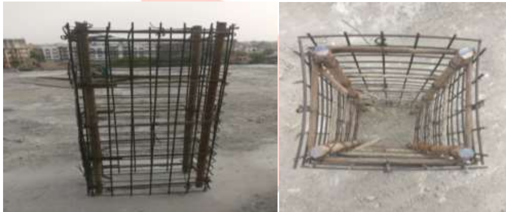
Fig.3. Reinforcement binding with welded wire mesh for rectangular column.
