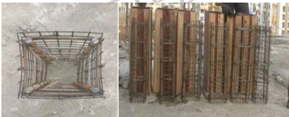
Fig.4 Reinforcement binding with welded wire mesh for Square column.
